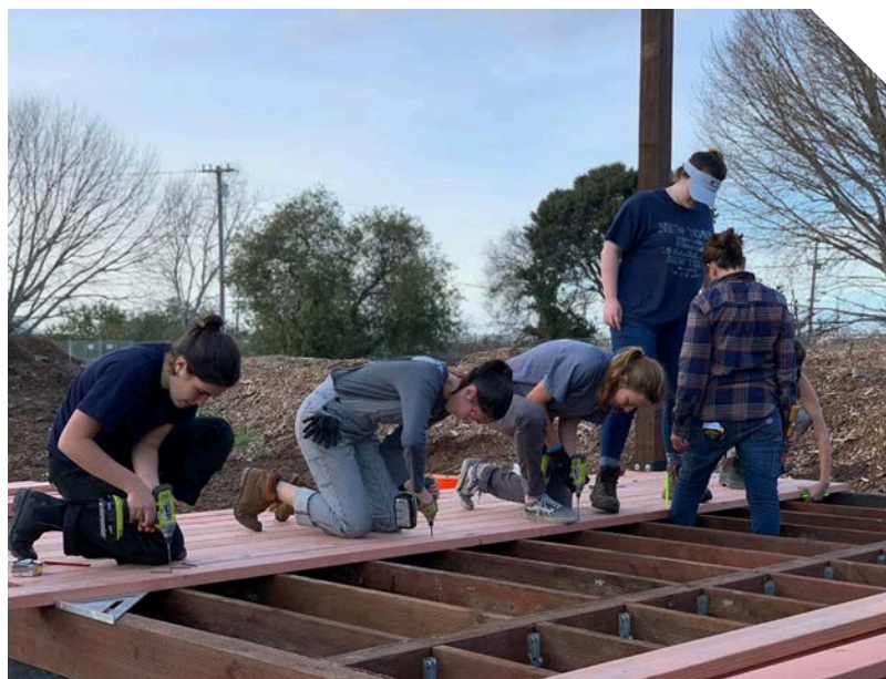
LAYING REDWOOD DECKING FOR THE CHICKEN COOP STRUCTURE AT URBAN TILTH DECEMBER 2019
