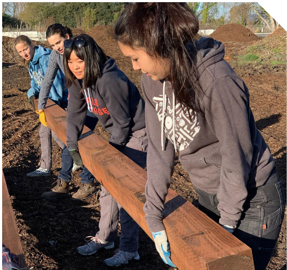
CURRENTLY BUILDING A LARGE CHICKEN COOP FOR URBAN TILTH, A LOCAL COMMUNITY FARM SEPTEMBER 2019
